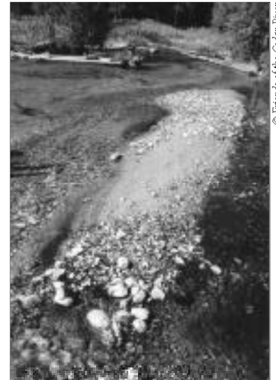
In August 1998, rainstorms washed hundreds of tons of soil, gravel, and turf chemicals from a new riverfront golf resort into Antrim County's Cedar River, which is not currently protected by Michigan's Natural River Program.
