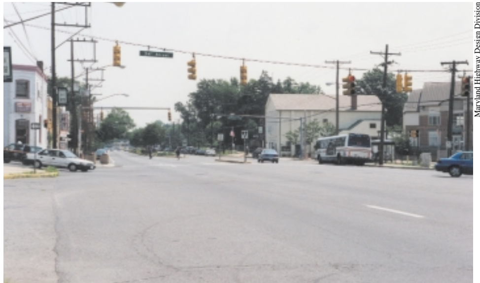
A six-way intersection in Mount Rainier, Maryland, known locally as the “sea of asphalt,” stymied all attempts at commercial revitalization until it was replaced with a traffic roundabout.
